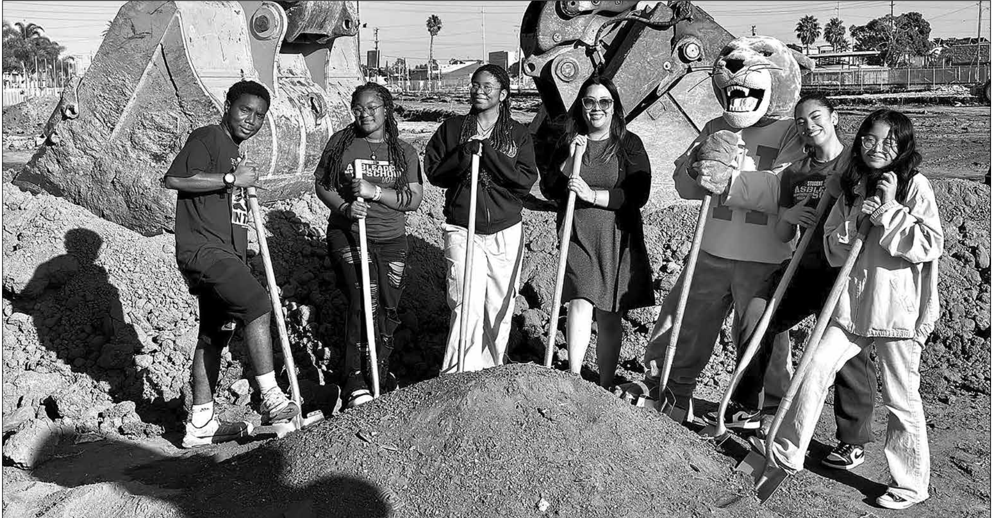
We celebrated the start of an exciting journey as we broke ground on the state-of-the-art Hawthorne High School Athletics Complex Project. Photo courtesy Centinela Valley Union High School District.
