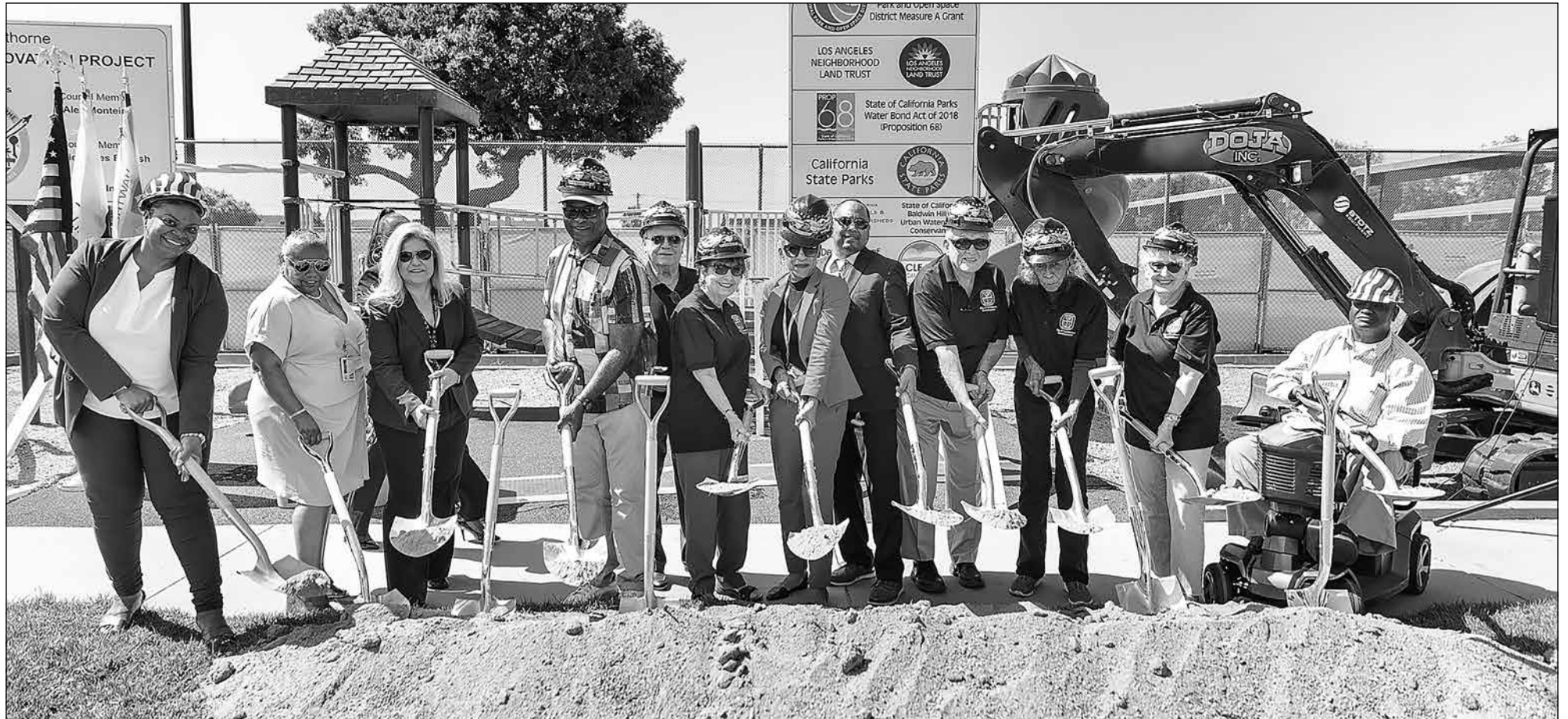
The City of Hawthorne and its Community Services Department had the pleasure of hosting a groundbreaking event for the Zela Davis Park Renovation Project. Hawthorne has received generous funding from several esteemed sources, including: Proposition 68, California State Parks, Clean California, Los Angeles County Regional Park and Open Space District and State of California Baldwin Hills Urban Watersheds Conservancy. Their support underscores the importance of the City's mission to enhance and revitalize our community parks for the benefit of all residents. Thank you for all your generous funding. Photo courtesy City of Hawthorne.
