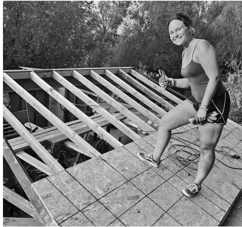
Lavelle "The Demolisher." Photos courtesy of Emily Lavelle.
