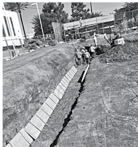
The crew works on the north area of the pool.
