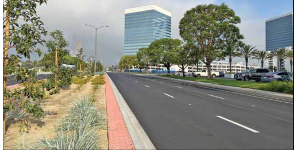
The El Segundo Boulevard Improvement Project was a significant infrastructure initiative that enhanced road safety and traffic flow. Photo: City of El Segundo Public Works Department.
